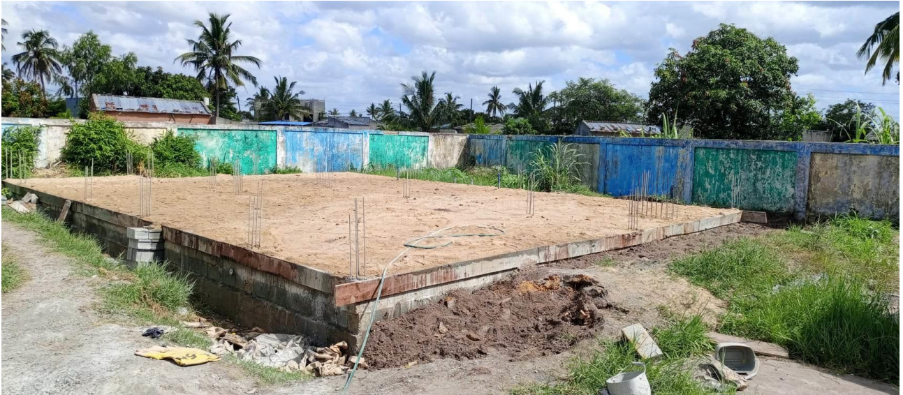
Completed foundations and base slab – November 2023
